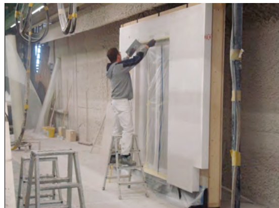
Applying a finish coat
