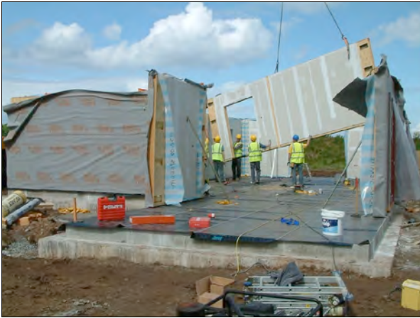
Day 1: ground floor panels are placed
