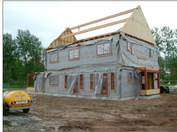
Day 3: Waiting for roof panels
