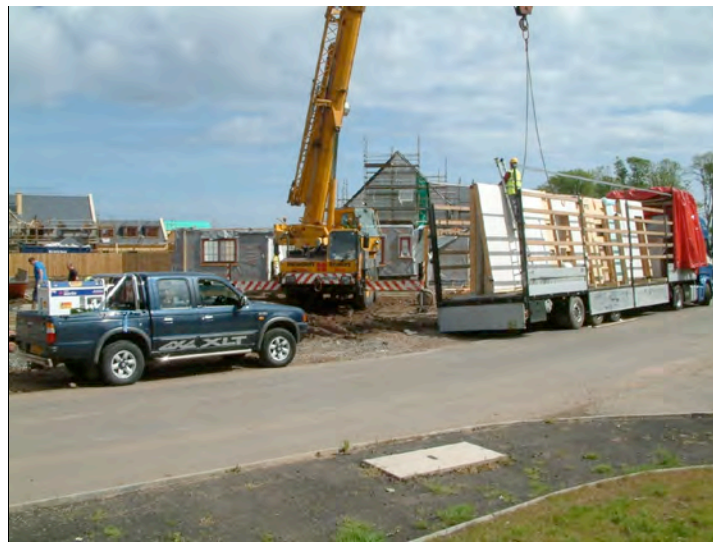
Panel hoisted from
