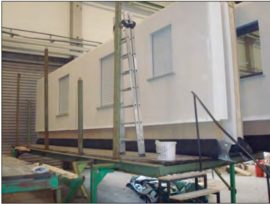
Panels ready to be placed on steel decks for transportation
