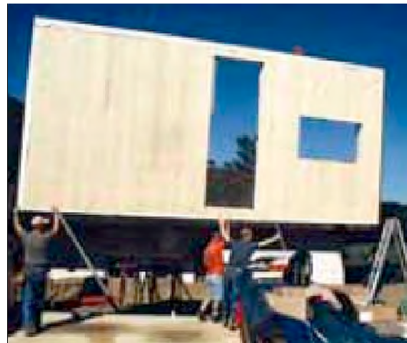
Placing a panel
