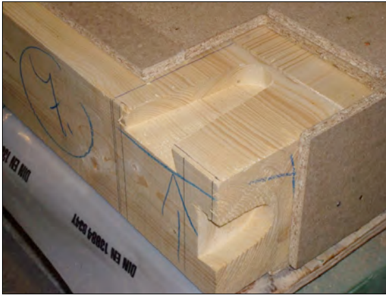
Dovetail Mortise (left) and Tenon (right)
