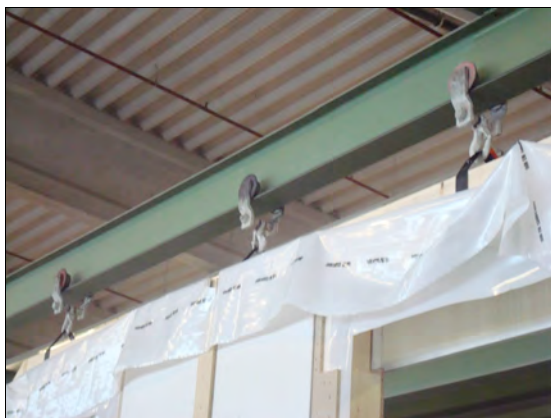
Panels suspended from rail by straps
