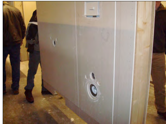
Precut cutouts in plasterboard
